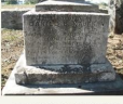
The black you see usually isn't dirt, it's biological growths, and can be lightened without any scrubbing
