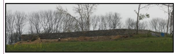
Left: front view after trees were removed and shredded and the front wall was repaired and re pointed.
